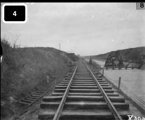
IWM / Q. 47161 / Achiet-Marcoing Line - Hermies Diversion. Track laid along tow-path of Canal du Nord.
