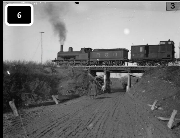
IWM / Q 47153 / Achiet-Marcoing Line. Bridge over Velu - Morchies Road. 26. 11. 17. Map Ref. Sheet 57C. I. 30. b.
