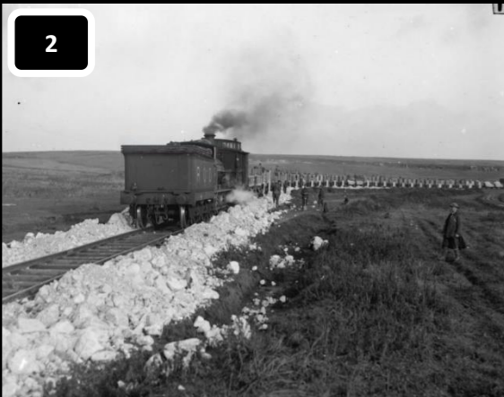
IWM / Q 47158 / Achiet-Marcoing Line (Hermies Diversion). Ballast Train being unloaded.
