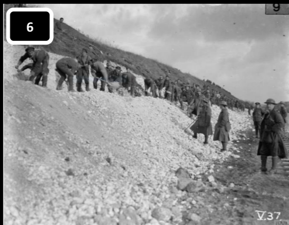
IWM / Q 47157 / Achiet-Marcoing Line (Hermies Diversion). Pioneers constructing grade. 22. 11. 17.
