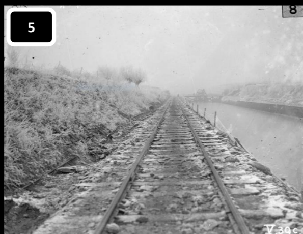
IWM / Q 47163 / Achiet-Marcoing Line (Hermies Diversion). Completed track along tow-path of Nord Canal. 19. 12. 17. Map Ref. Sheet 57. C. J. 36.
