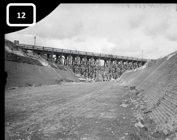
IWM / Q 47510 / Achiet-Marcoing Line, (Hermies Diversion). Bridge over Nord Canal.
