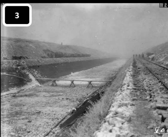
IWM / Q 47164 / Achiet-Marcoing Line (Hermies Diversion), Completed B. G. track along tow-path of Canal and Light Railway Construction Party at work on opposite side. 20. 12. 17. Map Ref. Sheet 57. C. K. 31.
