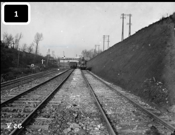
IWM / Q 47144 / Albert - Arras Line. Deep cutting for doubling of Achiet-le-Grand - Bapaume section of Achiet-Marcoing Line, near Achiet-le-Grand Junction; 26. 11. 17. Map Ref. Sheet 57C. G. 10. 6.
