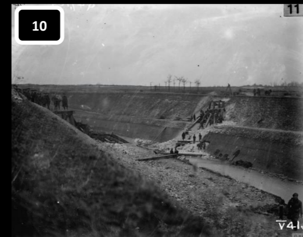
IWM / Q 47169 / Achiet-Marcoing Line (Hermies Diversion). Trestle Bridge carrying line over Nord Canal, under construction. 27. 11. 17. Map Ref. Sheet 57C. K. 26. C
