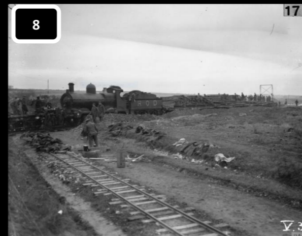
IWM / Q 47112 / Achiet-Marcoing Line (Hermies Diversion). C. O. R. C. Track Laying Train. 22. 11. 17.
